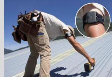
Smart PPE is worn by workers at the jobsite to provide real-time insight into physiological status. These wearables may collect data, adjust to conditions and warn of hazards. Algorithms created from that information provide an actional step for workers to take and allows an OSH professional to intervene when an injury or incident may occur.
